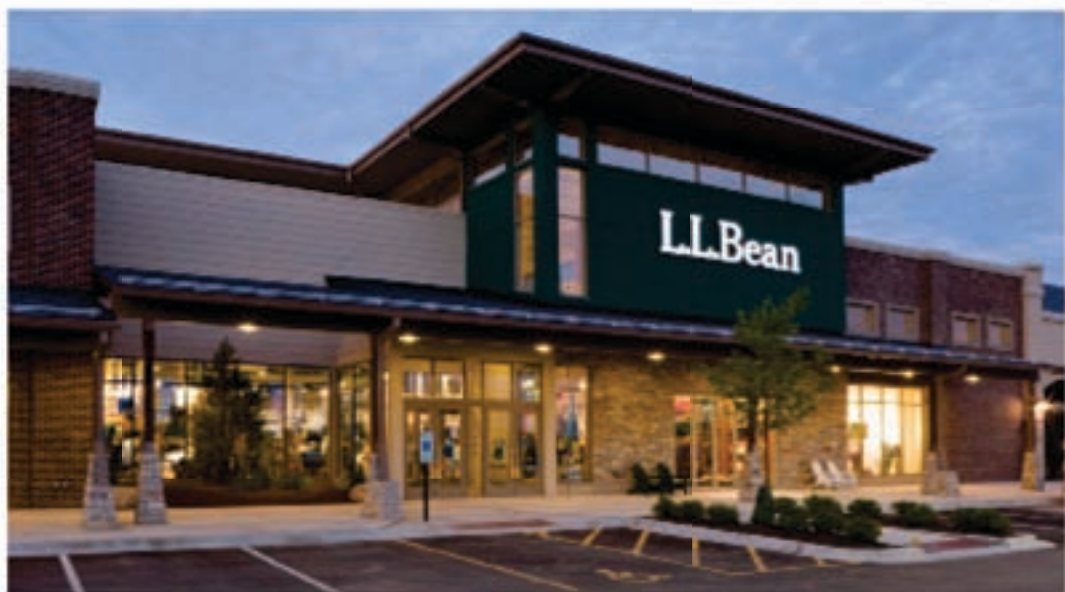
The L.L. Bean store at The Arboretum of South Barrington incorporates windows near the top for natural lighting and a white roof that reflects heat. The store also used recycled materials to build its fixtures.
