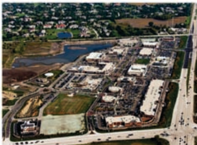
This aerial view of The Arboretum at South Barrington shows the large percentage of acreage devoted to responsible stormwater management.
